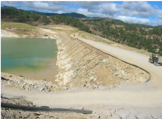
Upstream face with tailings spigot line
