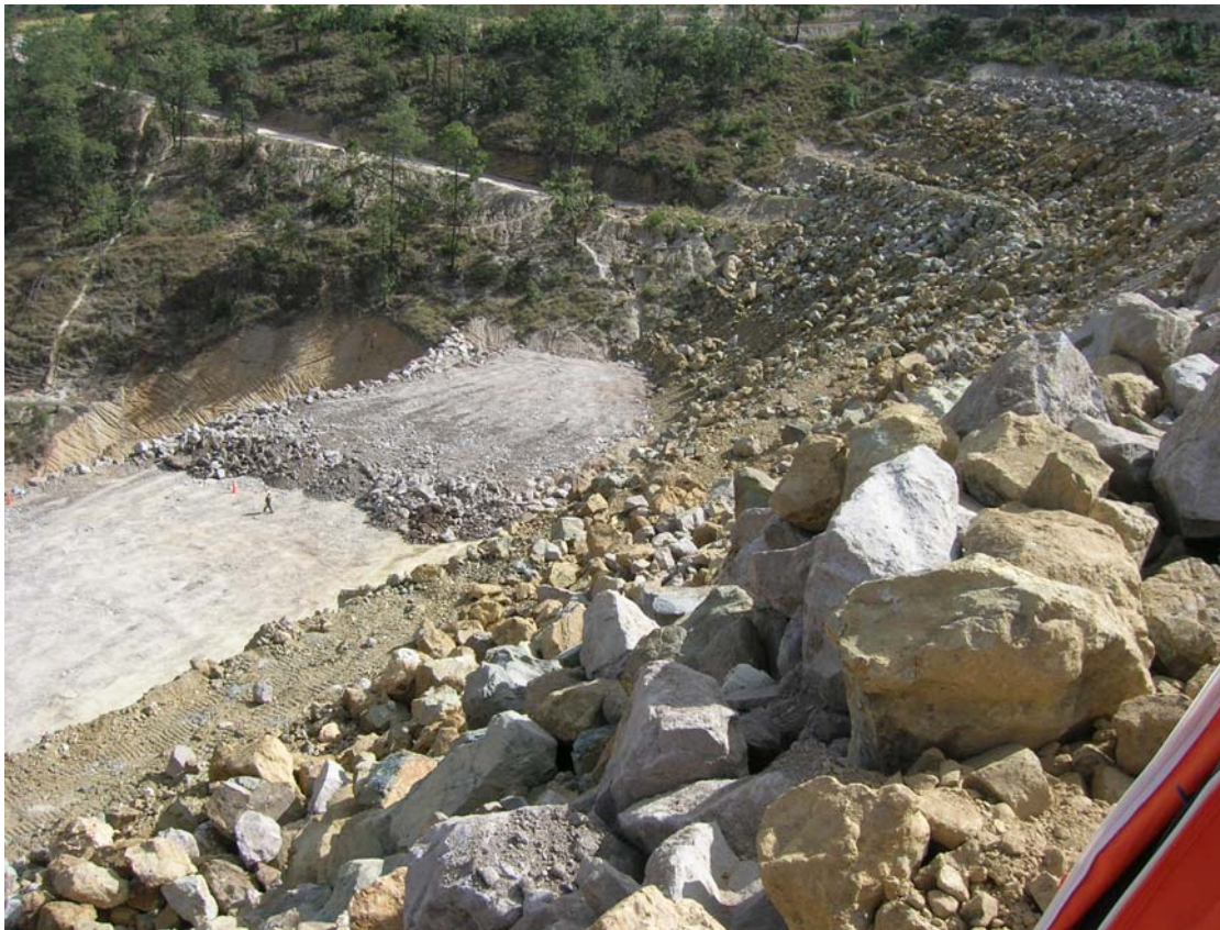
Photo 9 – Rockfill layer (grey) being placed on downstream shell zone
