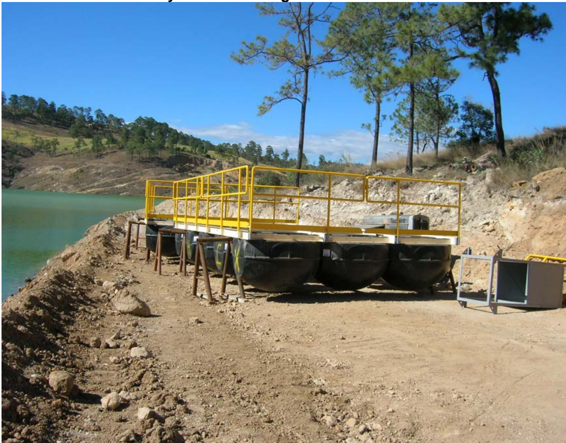
PHOTO 18 – Barge for replacement tailings water reclaim system
