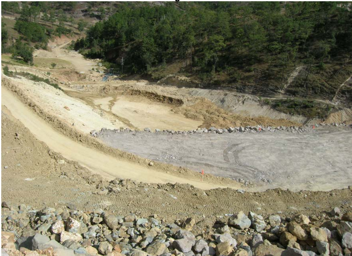
Photo 8 – Downstream toe showing Phase 2B raise rockfill (grey) over valley base under drain
