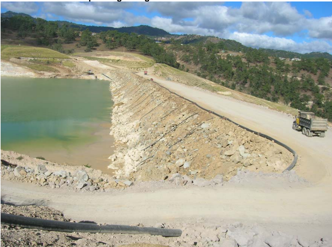
PHOTO 4 – Upstream crest (1948 m) of dam with tailings line and discharge spigots
