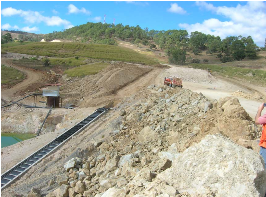
PHOTO 5 – Left abutment with stop-log decant sill set at 1939 (max 1942) with foundation preparation for construction of extension. Adjacent test tank for water treatment testing
