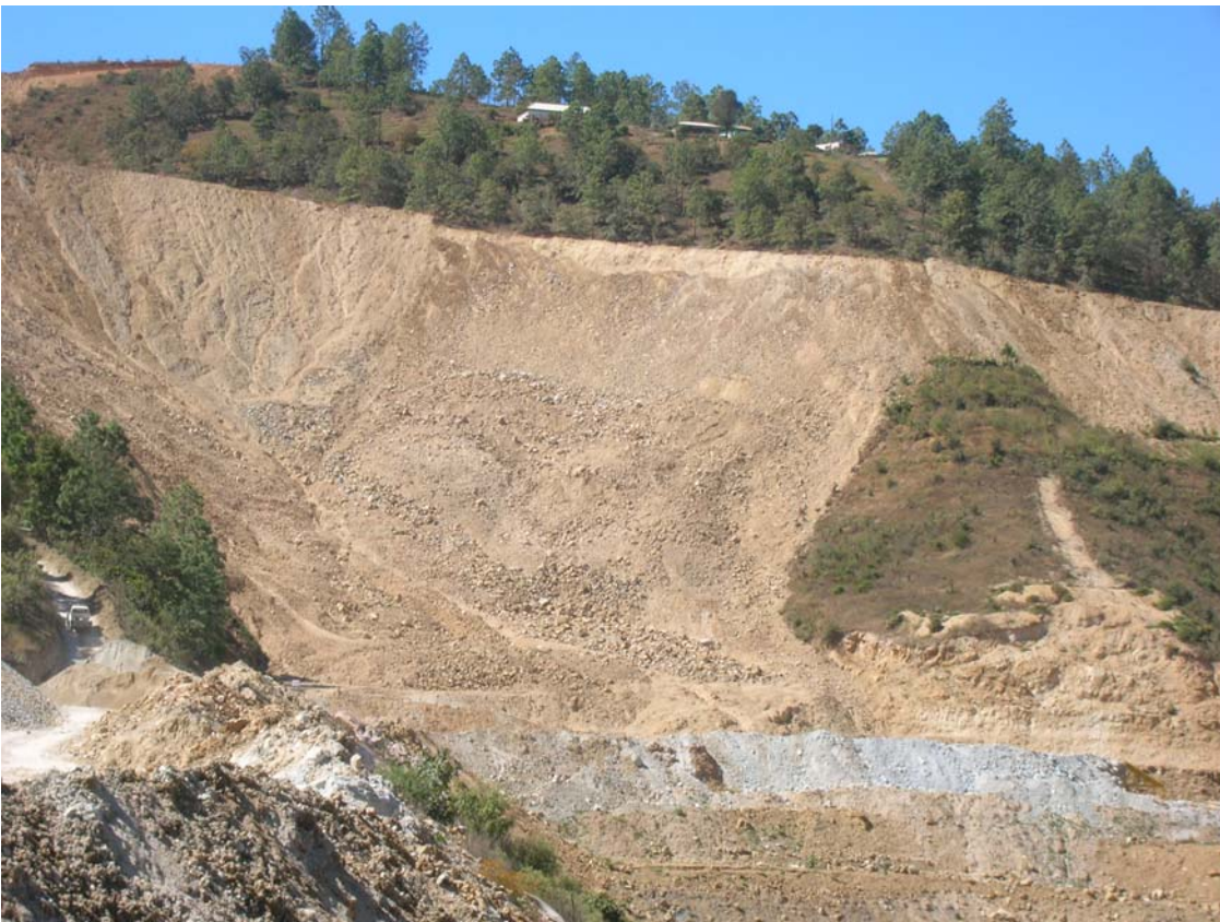
Photo 24 – Slump of waste rock slope on upper bench
