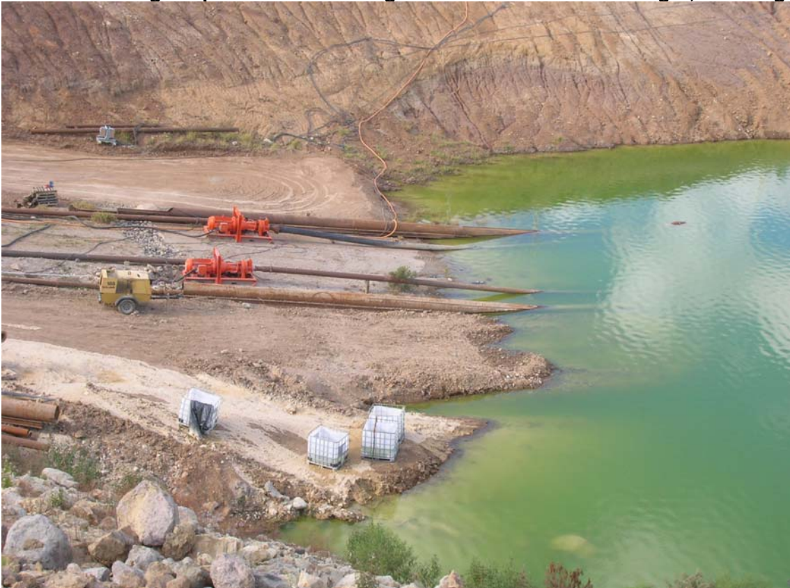
PHOTO 2 – Current tailings water reclaim pumps and intakes
