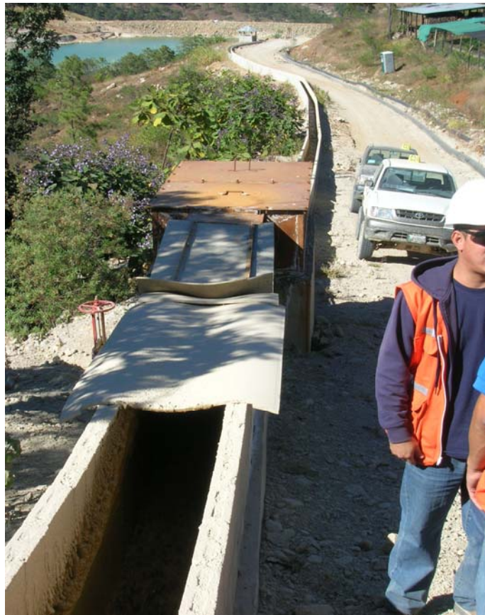
PHOTO 19 – Tailings flume with raised side walls and improved drop boxes
