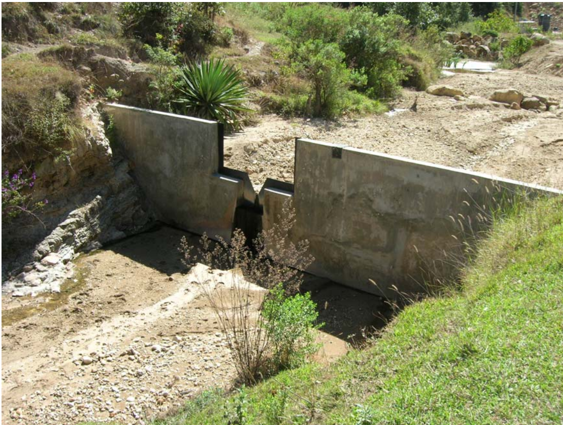
PHOTO 17 – Very low flow through V notch weir at d/s cut-off wall
