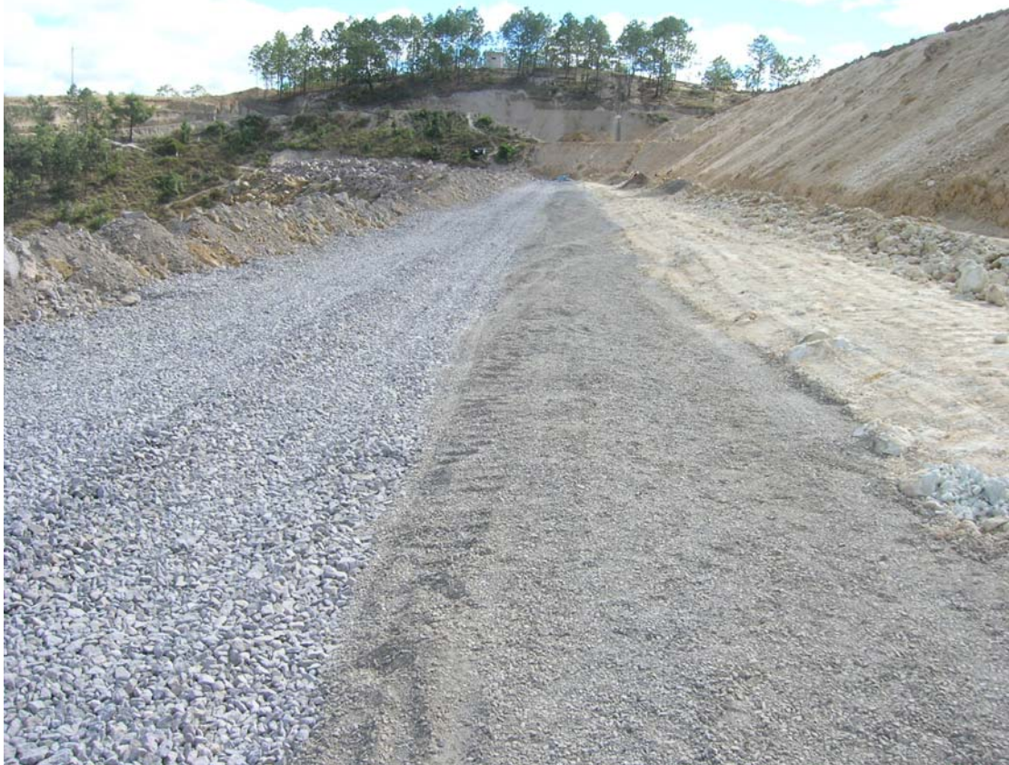
Photo 10 – Phase 2B core, fine filter and transition zone on bench ahead of d/s shell
