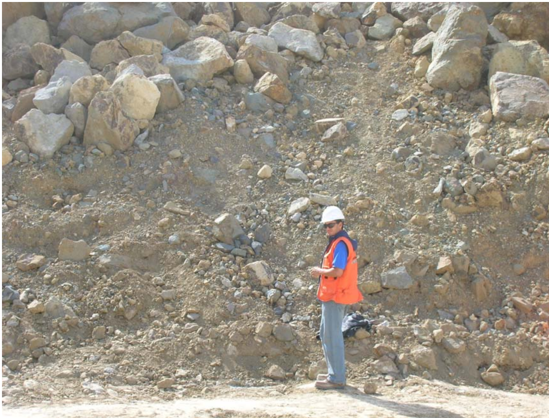
PHOTO 13 – Typical d/s shell fill after stripping of surface boulders
