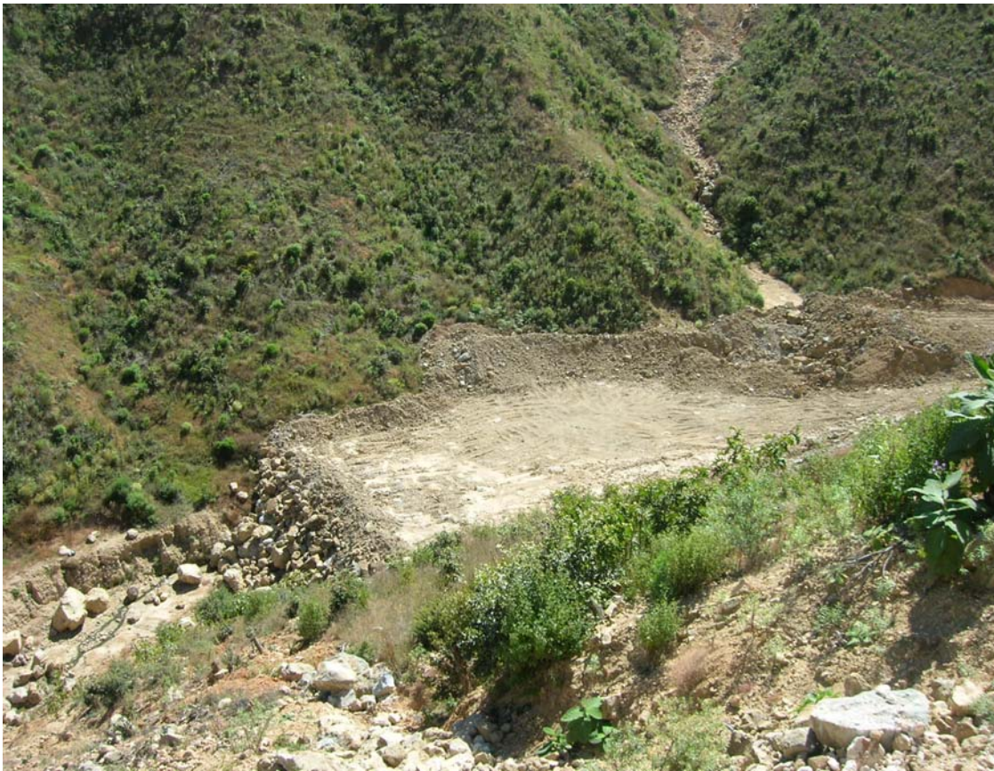
PHOTO 23 – Toe drain for WRF
