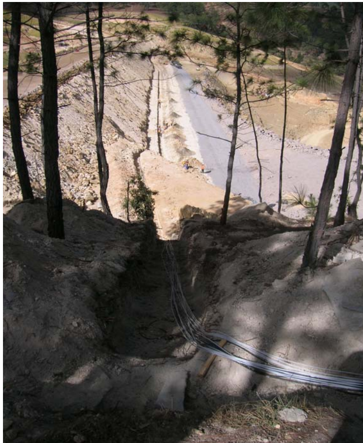
PHOTO 11 – Trench in core zone carrying optical cables from piezometers
