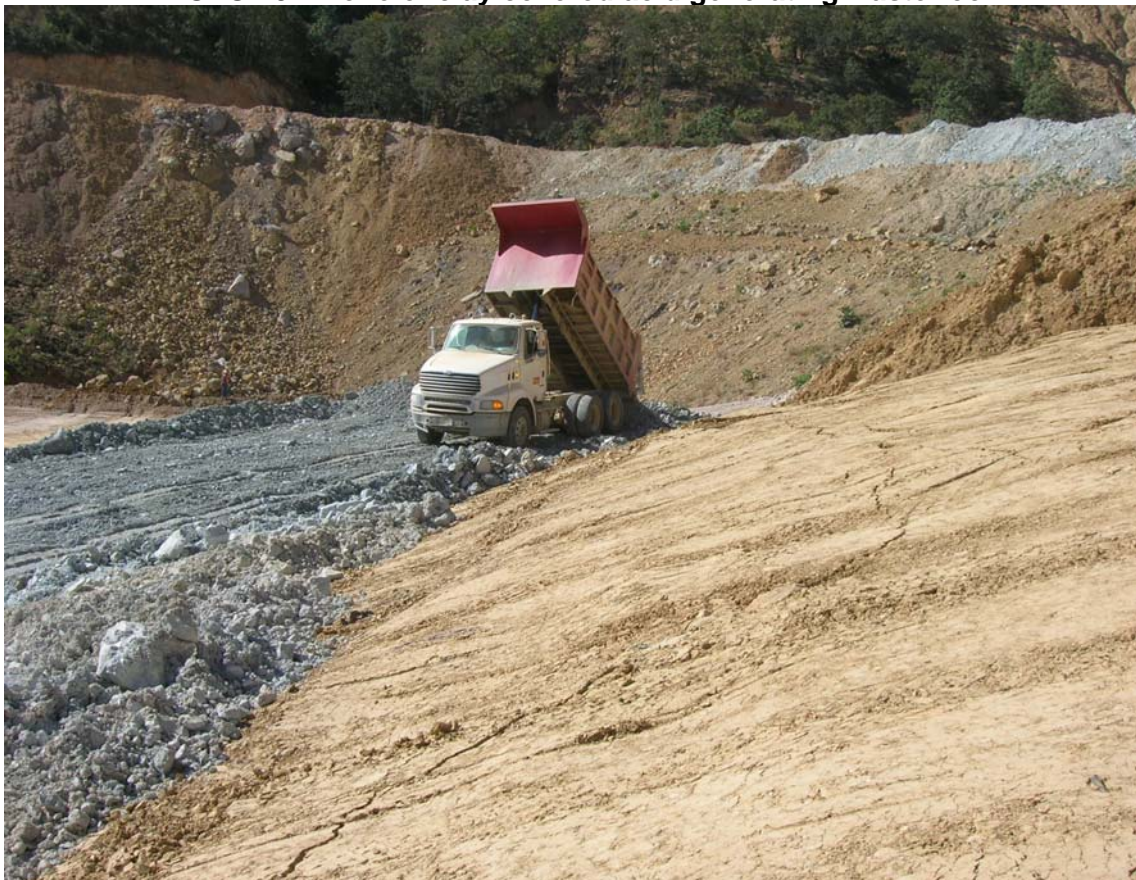
PHOTO 26 – Additional layer of ARD rock being placed. Note cracking of clay cover
