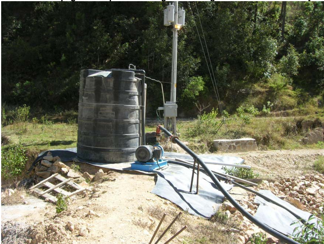
PHOTO 16 – New seepage return pump system
