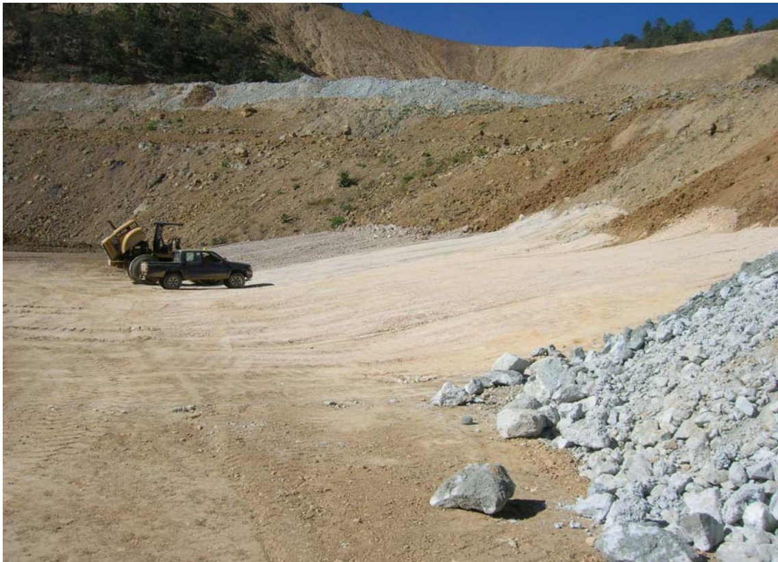
PHOTO 25 – Zone of clay covered acid generating waste rock
