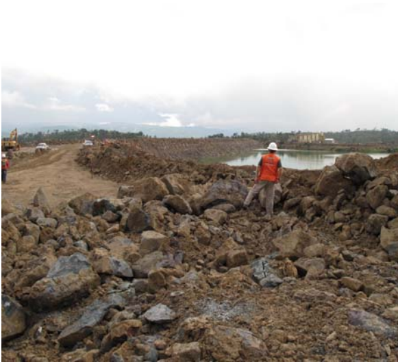
Tailings Dam crest at 1962 m, pond at 1949 m
