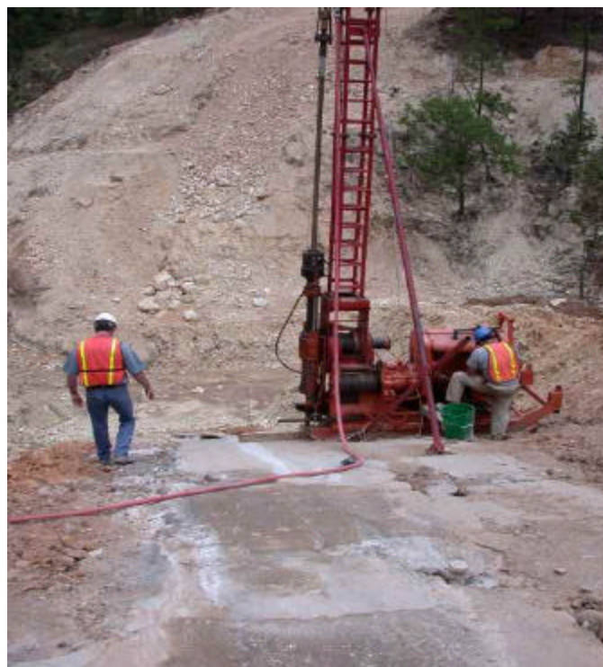
Photo B-2: July 12, 2004, Grouting on Right Abutment
