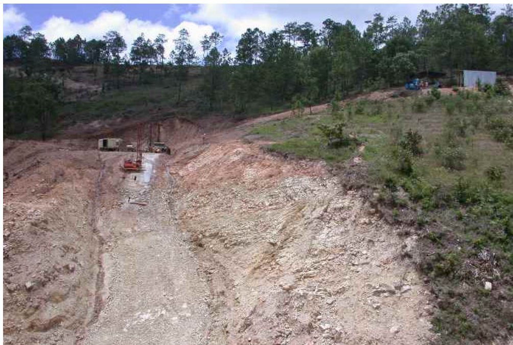
Photo B-4: July 12, 2004 Right Abutment Core Trench Excavation
