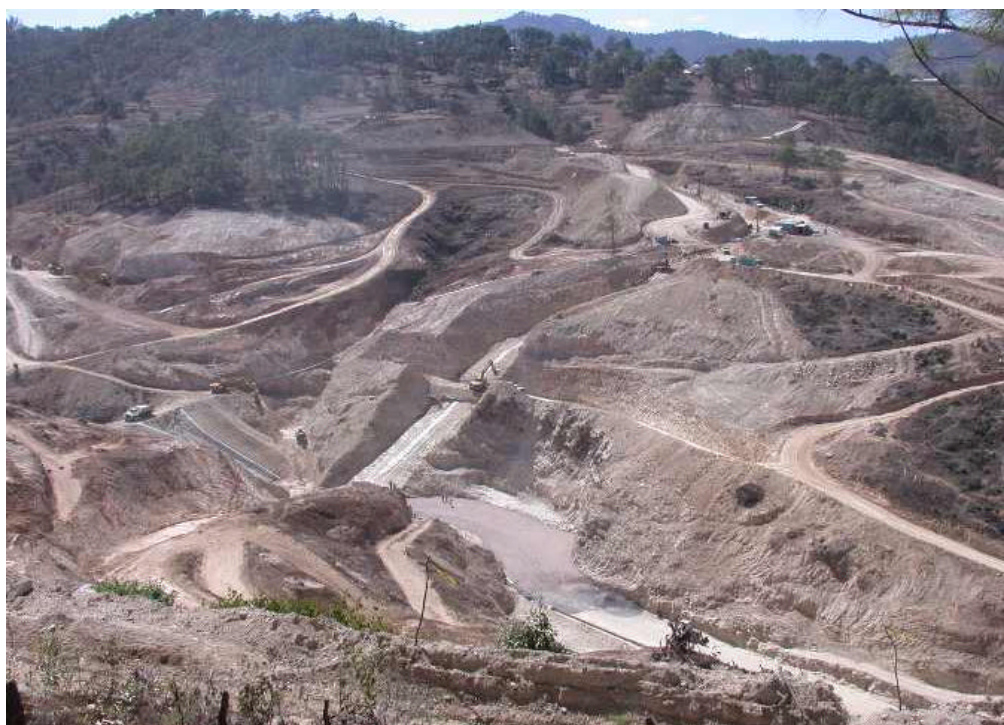
Photo C-4: February 21/22, 2004, Left Abutment excavation
