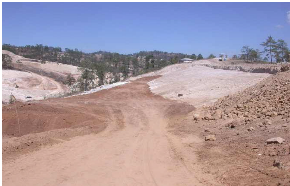
Photo C-14: Initial Core Placement for Saddle Dam on East Flank
