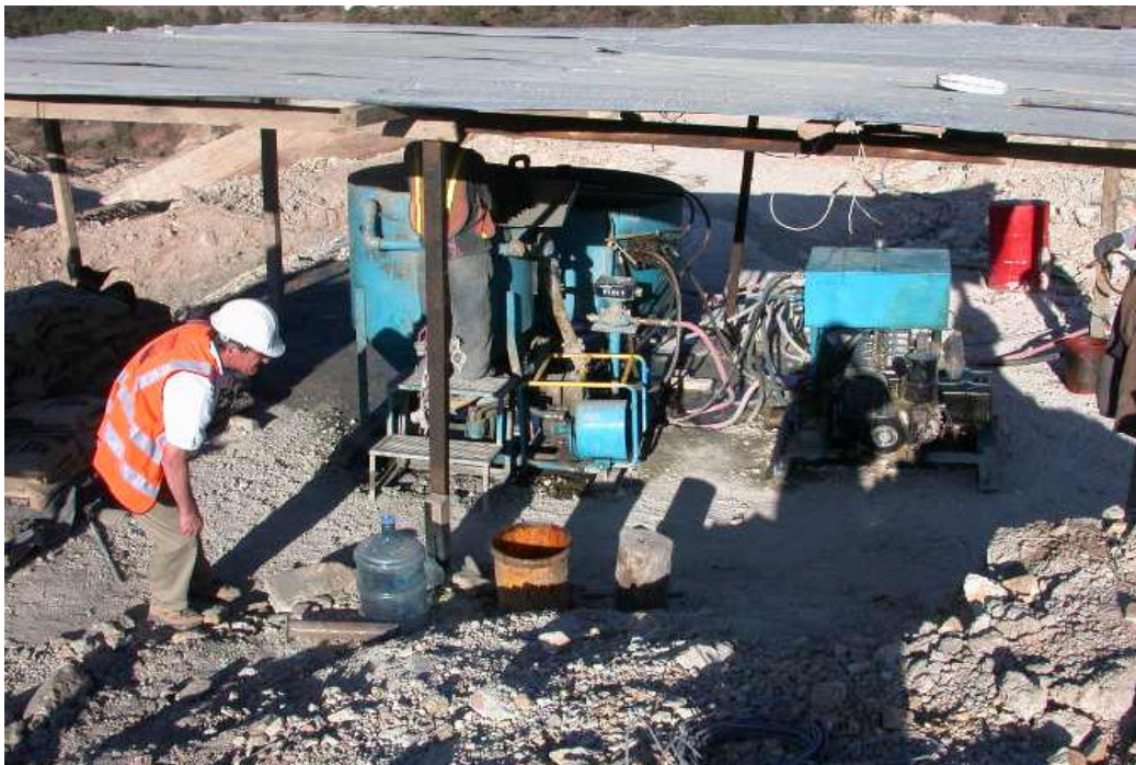
Photo C-7: February 21/22, 2004, Grouting Mixer and Pump
